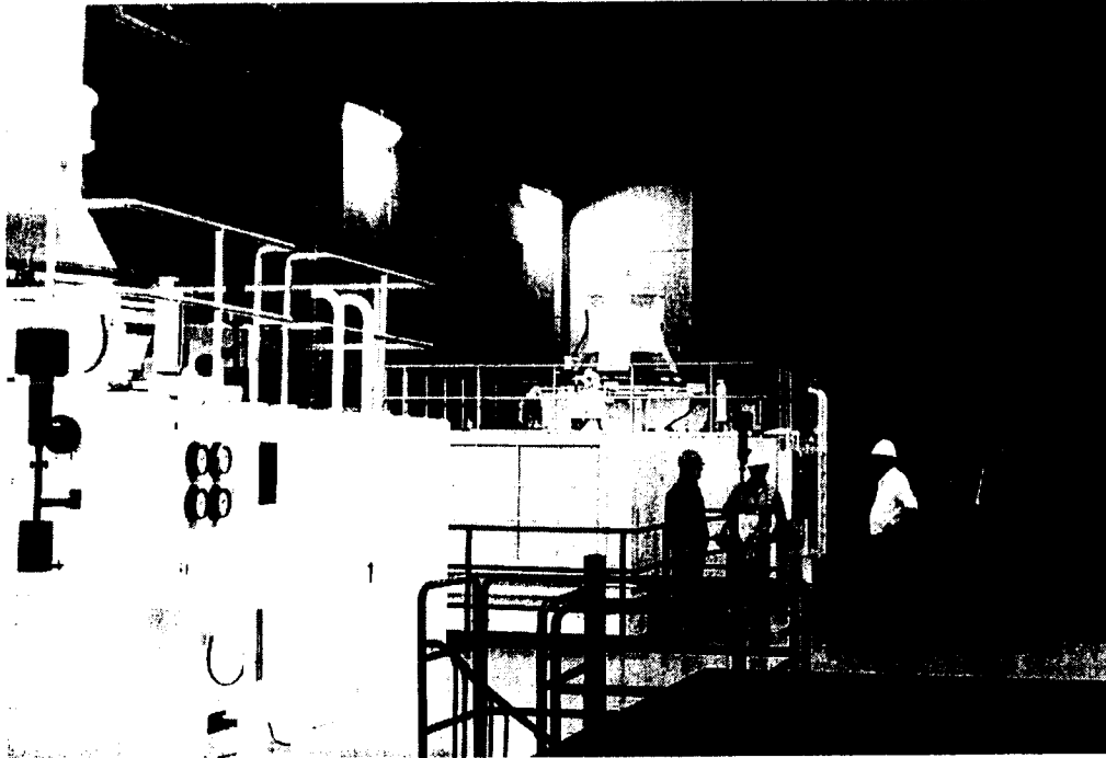
FIGURE 10.31. Deep tunnel pumping station in Chicago, Illinois. (Photo: V. Novotny.)
