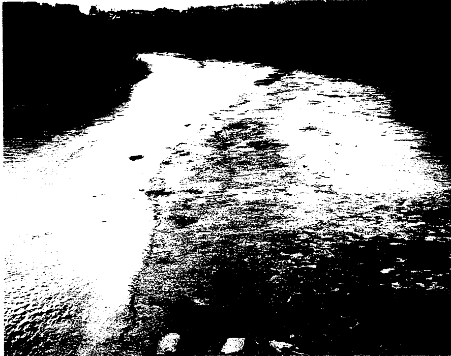
FIGURE 15.10. North Avenue impoundment on the Milwaukee River immediately after drawdown with exposed mudflats. (Photo: W. Wawrzyn, Wisconsin Department of Natural Resources.)
