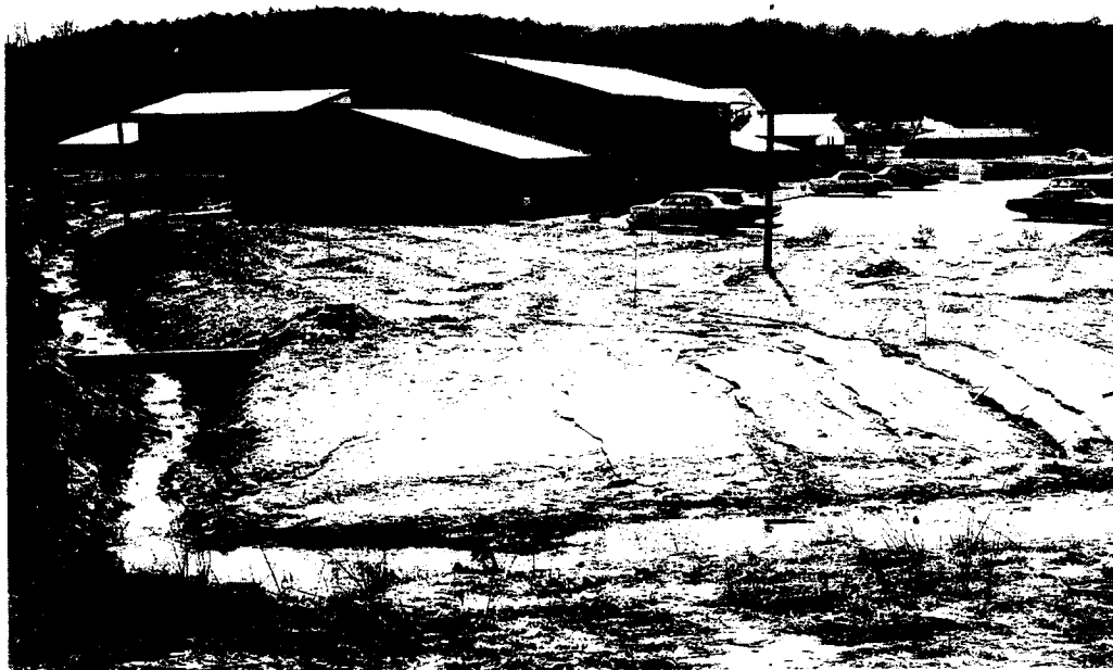
FIGURE 5.3. Sheet erosion of construction sites. (Photo: USDA—SCS.)
