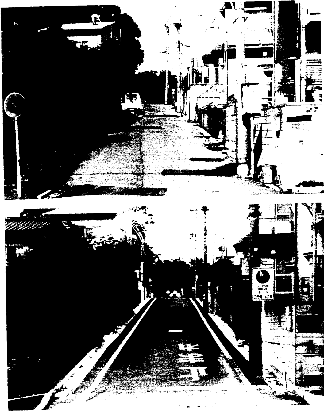
FIGURE 10.8. Example of porous pavement installation in an experimental basin in the Tokyo metropolitan area. Before ( top ) and after ( bottom ) installation. (Photo: S. Fujita.)
