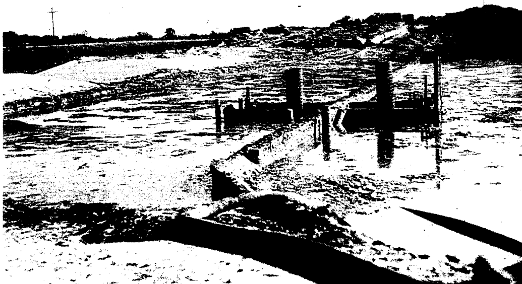
FIGURE 11.12. Large two-stage lagoon for containment of dairy animal waste. The first stage provides solids separation. (Photo: S. Alexander.)
