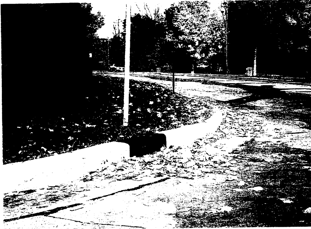
FIGURE 8.5. Leaf fallout in urban areas and its washoff into storm sewers is a source of large urban loads of biodegradable organics. (Photo: V. Novotny.)
