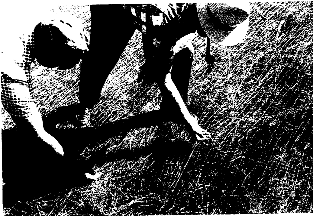
FIGURE 10.5. Mulch net applied over straw mulch, seed, and fertilizer. The net is of paper fiber with plastic strands that are pinned down over the straw. (Photo: USDA, Soil Conservation Service.)
