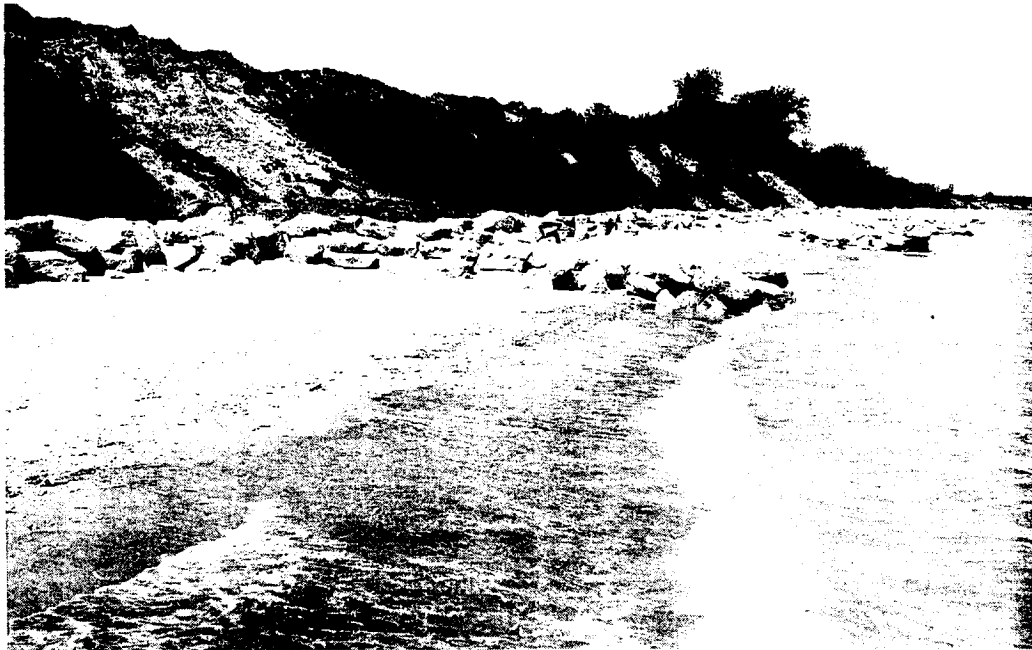
FIGURE 5.6. Shoreline erosion. (Photo: V. Novotny.)
