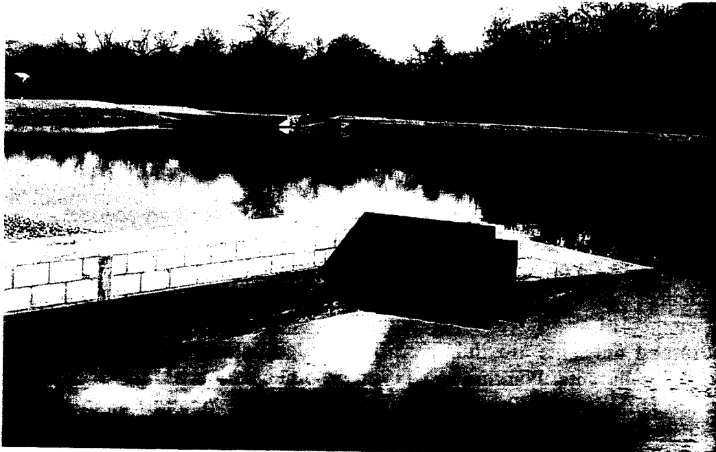
FIGURE 11.10. Retention pond—sedimentation basin. (Photo: S. Alexander.)
