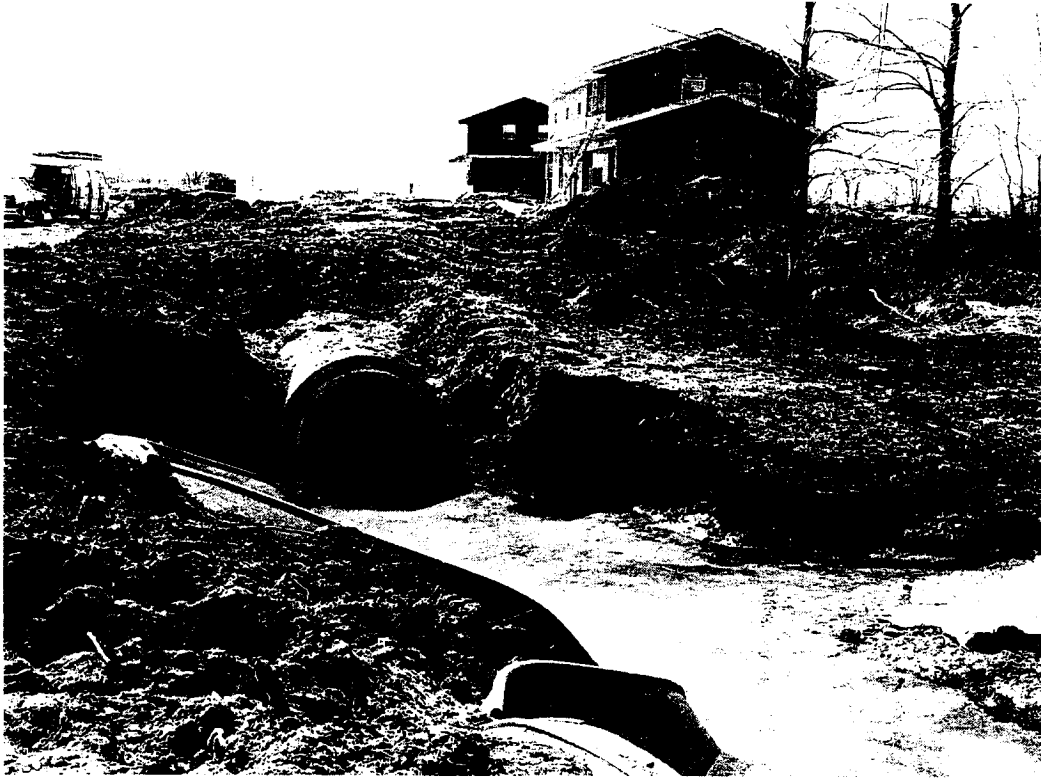
FIGURE 10.14. Erosion of unprotected channels in construction zones. (Photo: University of Wisconsin.)
