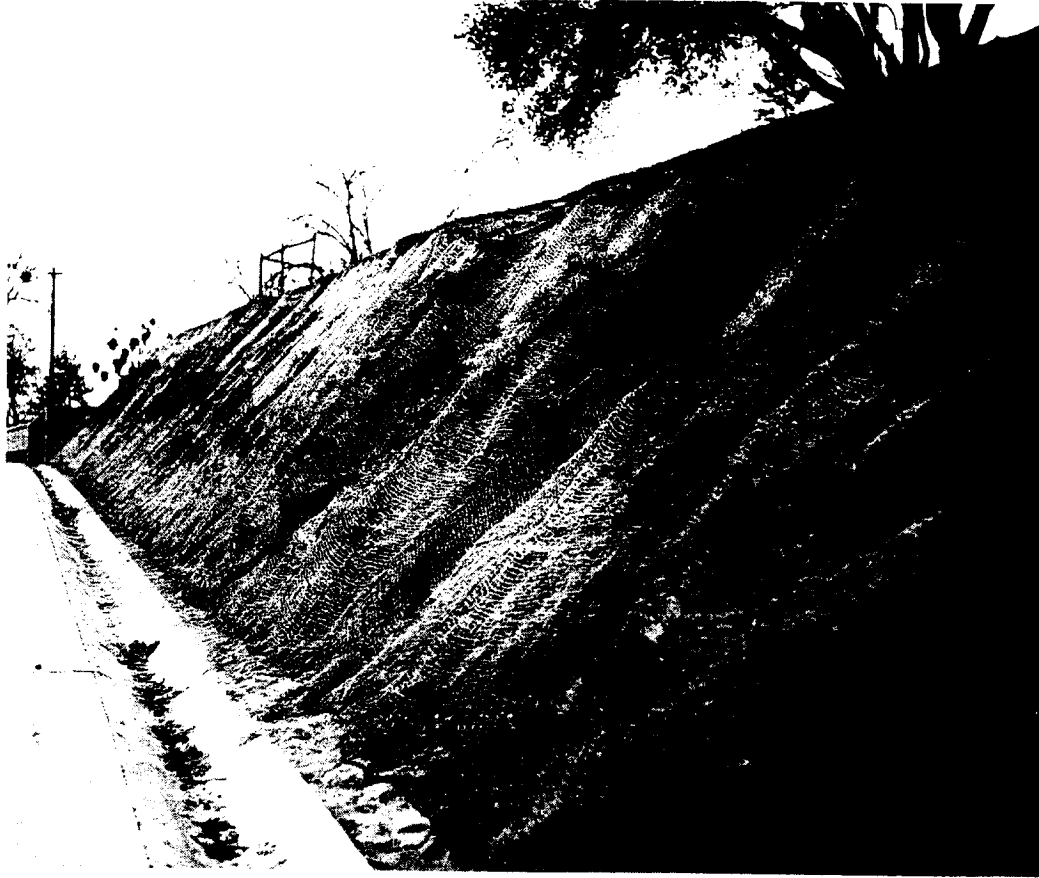
FIGURE 10.6. Control of erosion by burlap netting. (Photo: USDA, Soil Conservation Service.)
